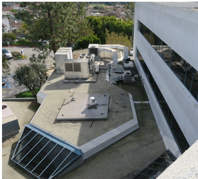
Fig 12 – 1976 MOB Exterior & X-Ray Roof
