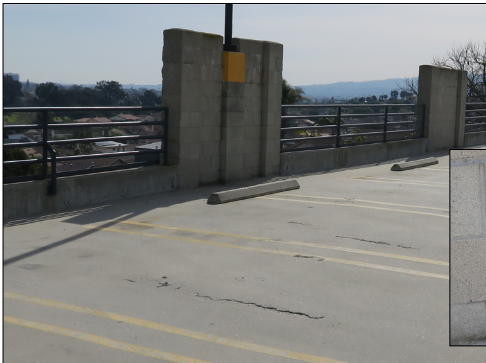
Figure 14 – Exposed Rebar, Parking Structure Top Deck; Narrow Masonry Piers and Spandrels
