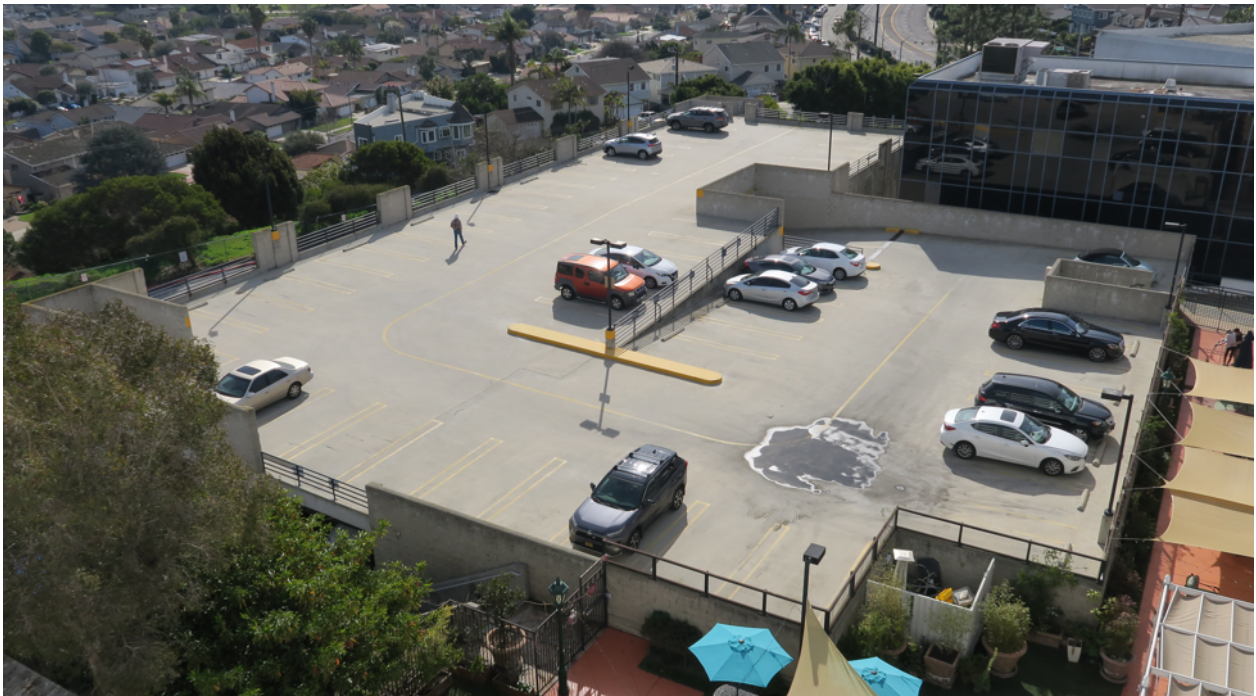
Figure 13 – Parking Structure Top Deck
